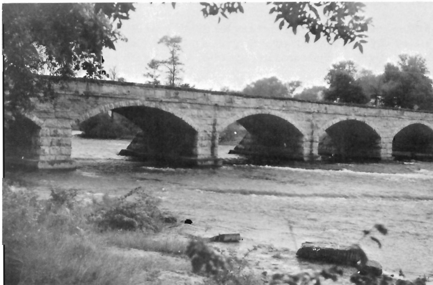
Plate I. Bridge over Mississippi River in Pakenham (GSC 153197).
