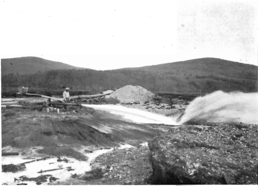
A. Stripping muck, frozen peat, and silt off of placer gravel with an hydraulic monitor.
