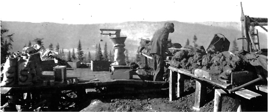
B. Sacking ore on the Hector group, Galena hill, 1935. The large lumps of galena seen in the picture are being broken up and sacked.
