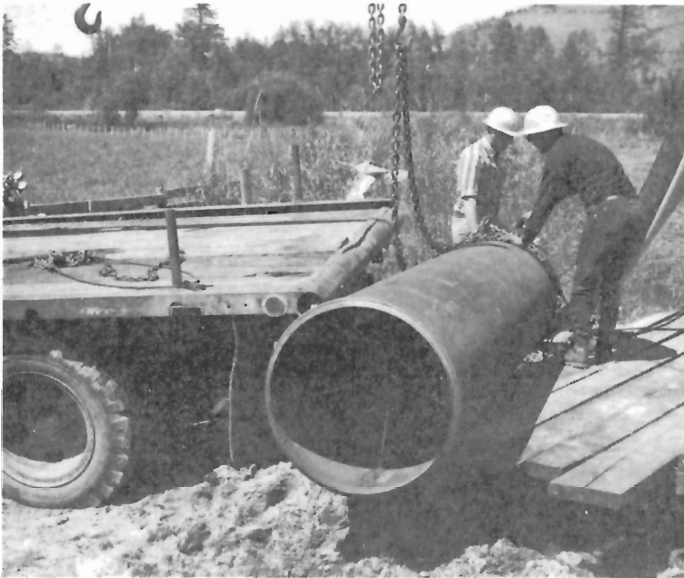
Figure 8. Guide shoe on initial length of 30 inch casing. GSC 125288.
