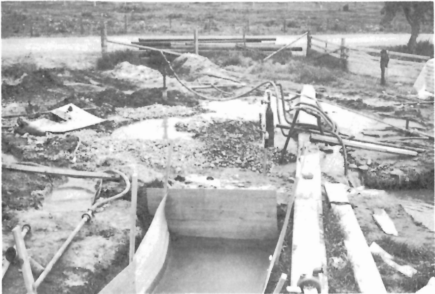
Figure 5. Mud sump and grout pipe installations, July 1965. GSC 118631.
