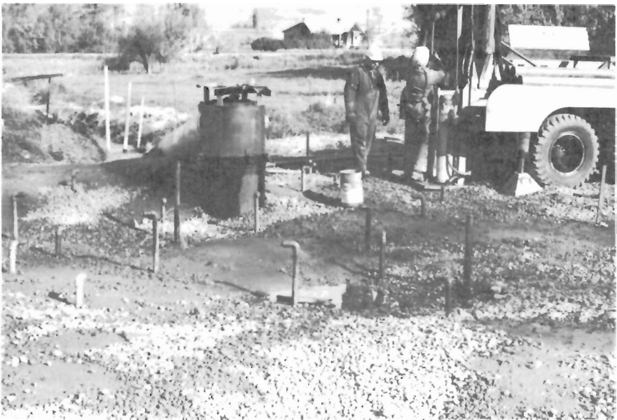
Figure 12. 1 1/2 inch diameter grout pipes installed in the crushed rock fill.
