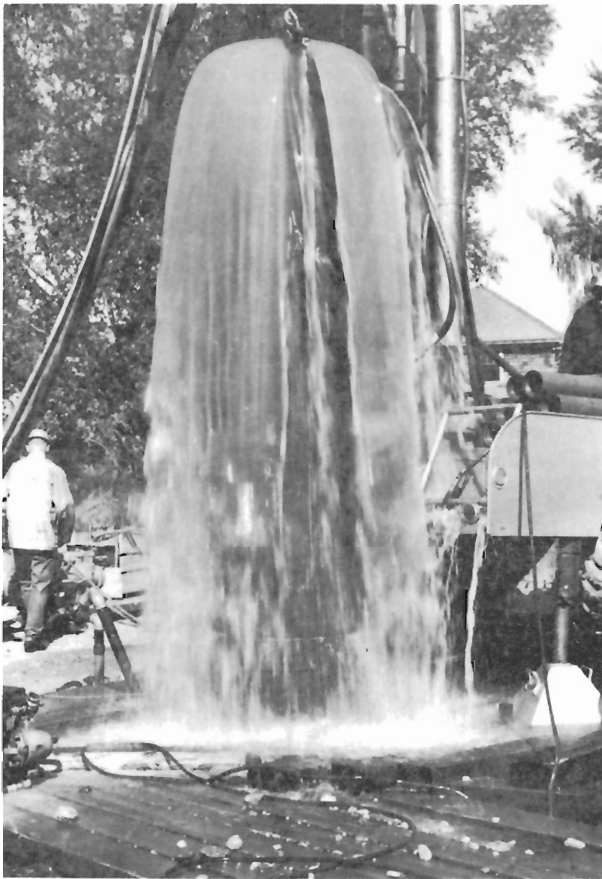
Figure 10. Full flow over the top of a 10 foot length of 30 inch casing. GSC 118661.
