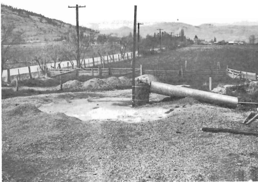
Figure 16. Well site upon completion of grouting crushed rock fill (April 1967). GSC 125296.
