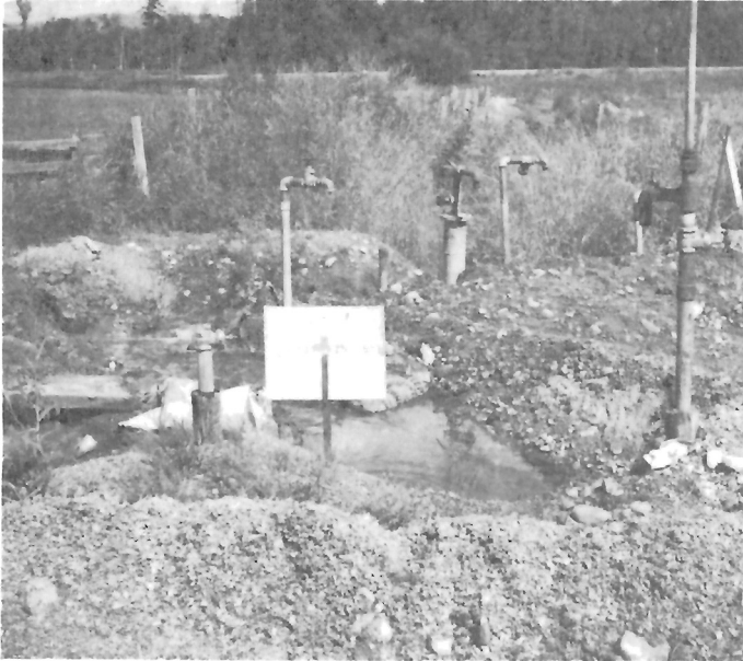
Figure 7. Cratered area in gravel fill at well site, July 1966. GSC 125295
