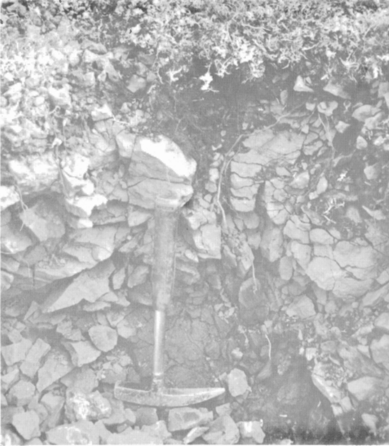
Figure A3. Breccia soil. (GSC photo 156835)
