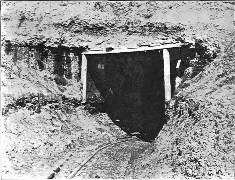
Entrance to mine of Superior Coal Company, north side of Belly river north of Taber, Alta. The hammer marks bottom of lignite seam underlain by shale, while the roof is sandy clay.
