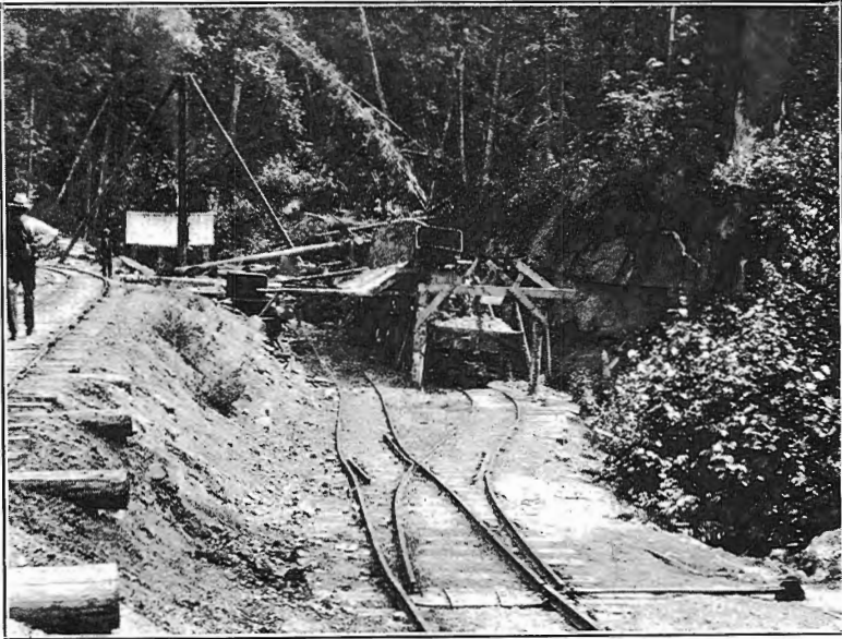
View looking up track of Clayburn Brick Co., Clayburn, B.C., showing entrance to mine which supplies the clay for buff brick. The section shown in Plate XXXV is on the left side of track.
