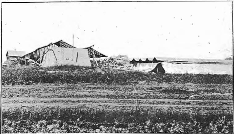
Brickyard at Saskatoon, Sask. Shows drying racks covered with canvas screens, to prevent too rapid drying and consequent cracking of the bricks.
